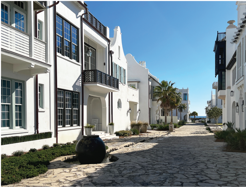
Figure 1. Alys Beach. This streetscape view of Alys Beach, Florida, illustrates the benefits of street orientation along a north-south axis because the buildings on the west side of the street shade the street throughout the afternoon. This location also aligns with southerly prevailing breezes and uses pervious paving, shaded entries, and white walls. Photo credit: DPZ CoDesign.
