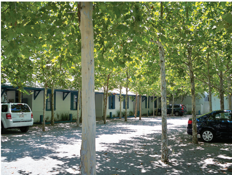
Figure 4. Seaside parking lot. This parking lot in Seaside, Florida, uses light-colored, pervious pavement and an allée of sycamore trees planted at distances that define parking spaces and reduce the heat load of a parking lot. Source: DPZ CoDesign.
