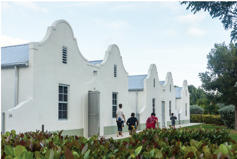
Figure 5. Blue water workforce housing. Blue Water Workforce Housing, Tavernier Key, Florida, illustrates the use of cool colors, reflective roofs, courtyards, and gardens positioned to enable cross-ventilation and plantings to shade the buildings. Source: DPZ CoDesign.
